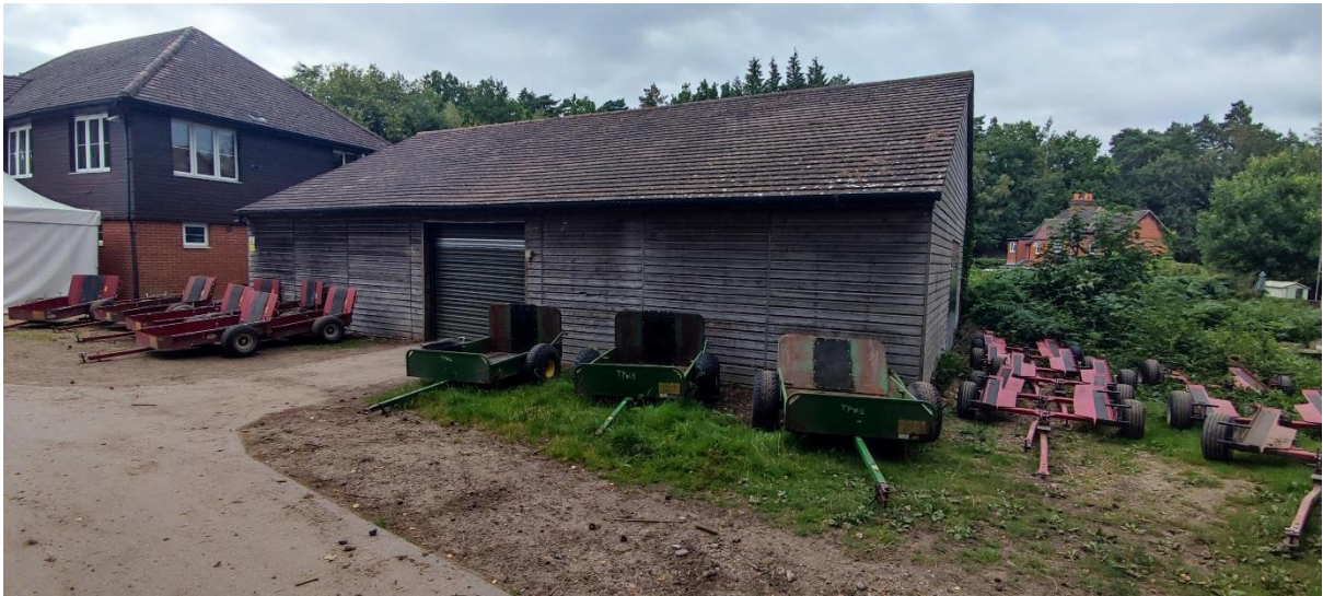
Storage building (to be demolished) adjacent to Building E (left)
