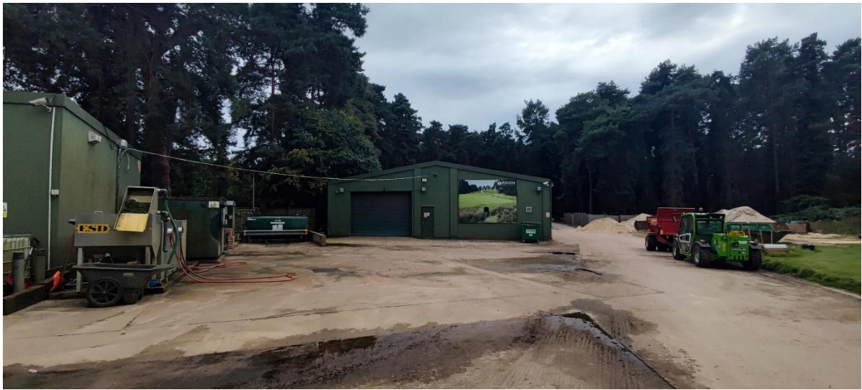
Existing building A (to be demolished)
